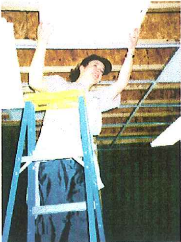
AmeriCorps Member hangs suspended ceiling.
